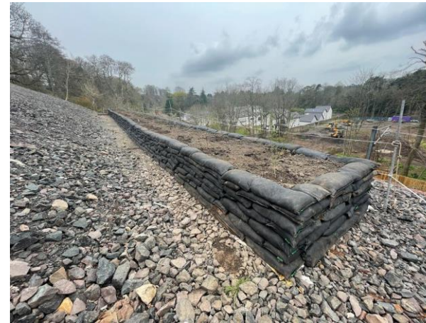
Raised beds installed as part of the Fairlie landslip remediation
