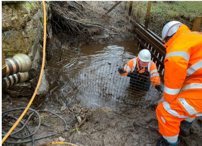
Construction of the Beaver pass at culvert near Gleneagles
