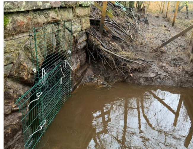
Constructed Beaver pass
