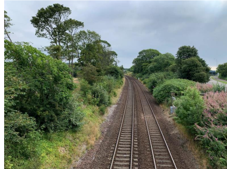
Dalgety Bay site after vegetation management works
